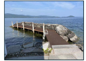
A view of the existing breakwater and cantilevered dock on Lake Winnepesaukee
