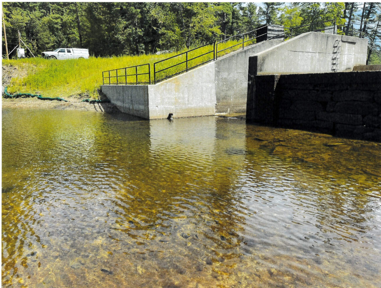
Photo 3: Looking east from left side towards power easement area. 8/2025
