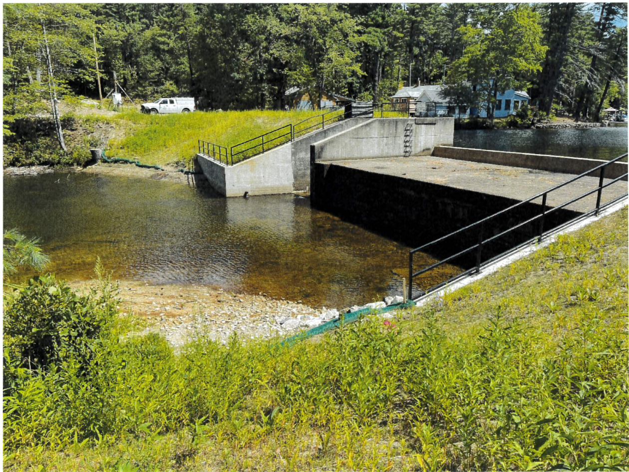
Photo 4: looking east from left side of dam towards easement area. 8/2025
