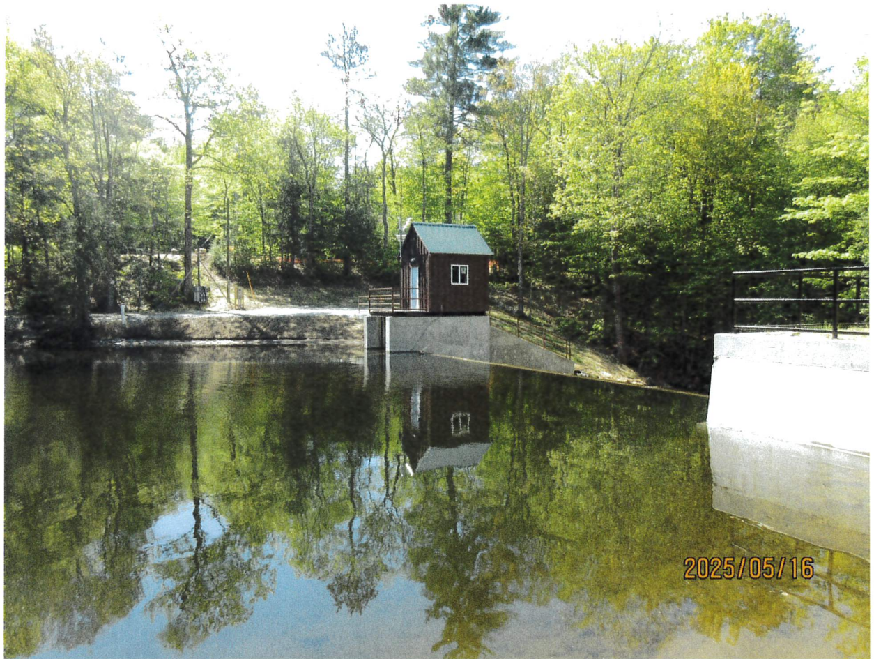
Photo 5: looking south upstream from right side of Dam. 5/16/2025
