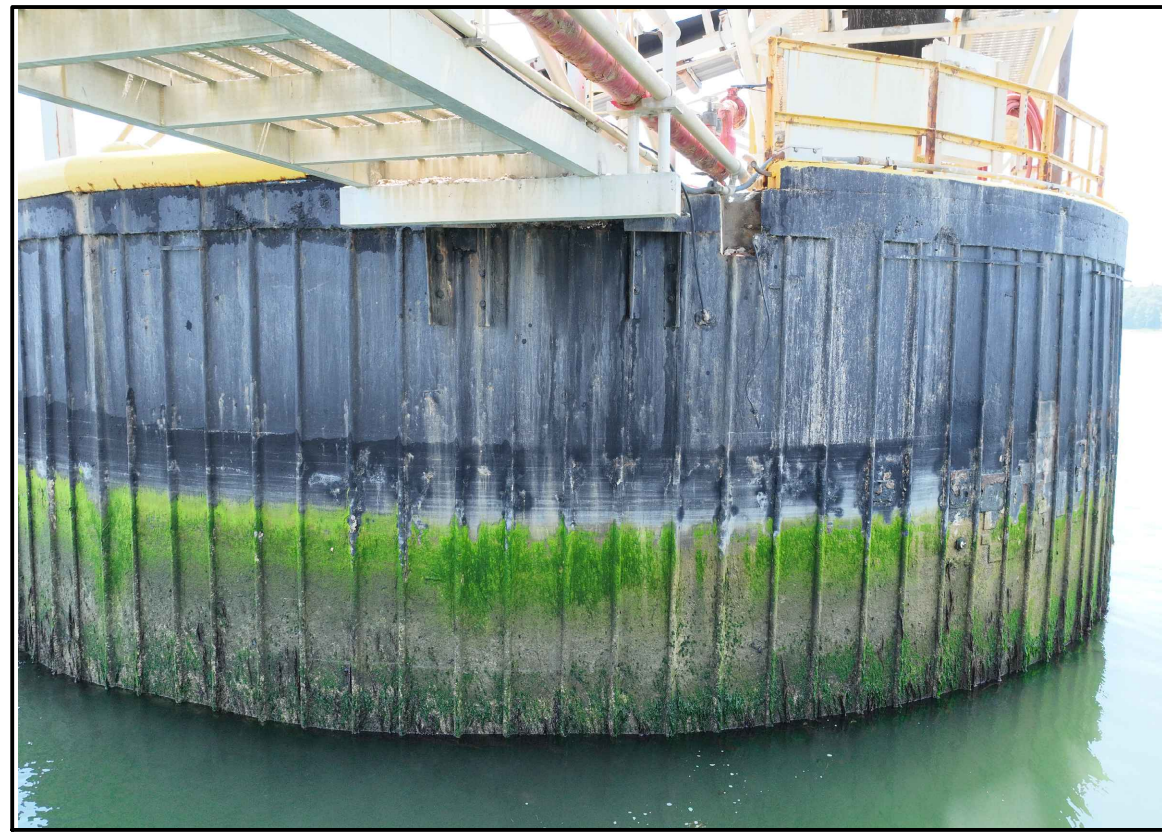
PHOTO 6 BERTHING CELL 2, LOOKING EAST SCALE: NTS C-001 B2
