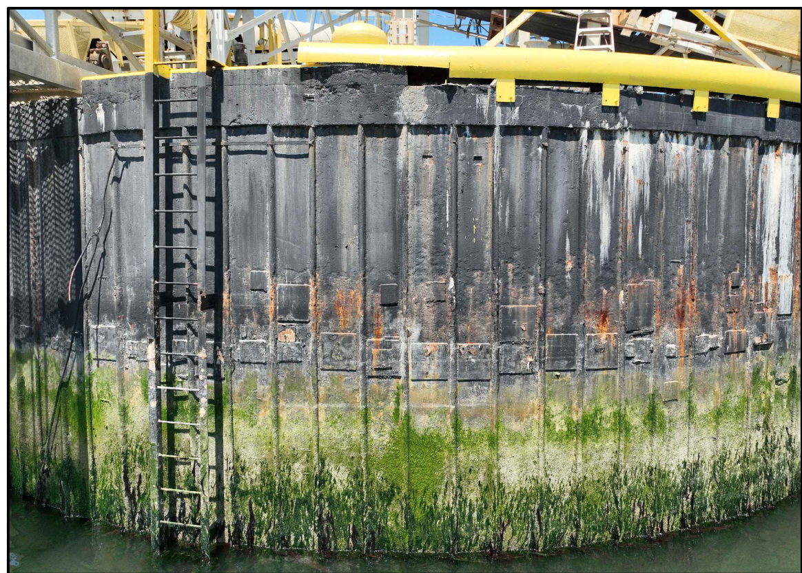
PHOTO 9 BERTHING CELL 2, LOOKING NORTHWEST SCALE: NTS C-001 A1
