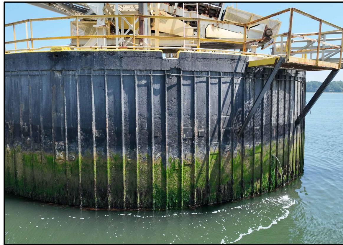
PHOTO 7 BERTHING CELL 2, LOOKING NORTHEAST SCALE: NTS C-001 B3
