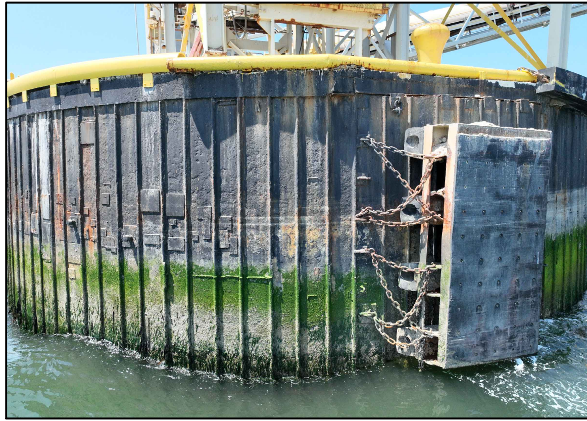
PHOTO 2 BERTHING CELL 2, LOOKING WEST SCALE: NTS C-001 C2
